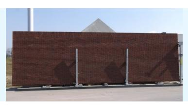
Walls higher than 4.25 meter generally have to be transported in a diagonal position. This is also supported by Blue Workx.
